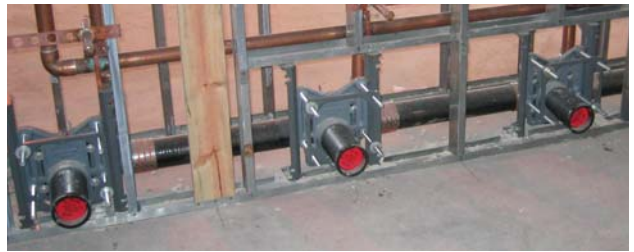
Prefabricating and installing the toilet carriers was easy. There are so many pipes in the ceiling that Grunau had to blow the plans up to one-quarter scale to see them all.
