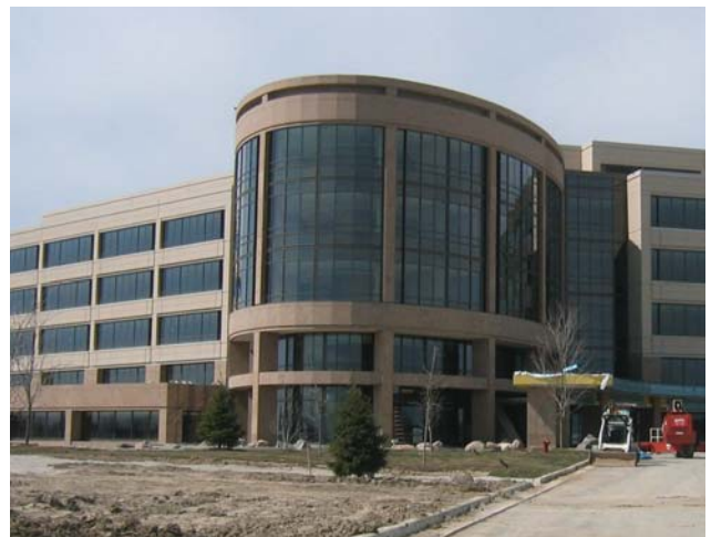
There is a free lunch at Northwestern Mutual and the huge first floor cafeteria with its water supply lines, floor drains and hub drains made the job a challenge for Grunau Co.
